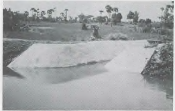
This newly concreted canal gate was part of the ADRA project.
