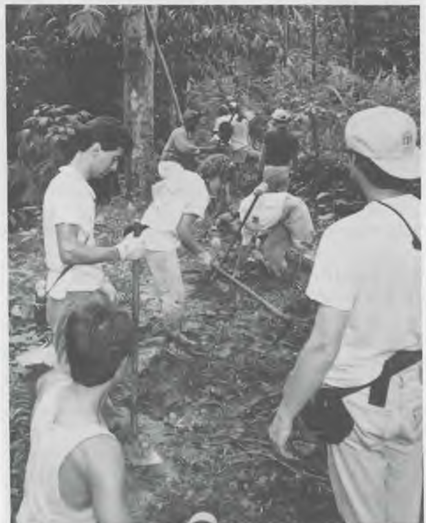
Volunteers help lay six kilometers of pipe through the jungle.
