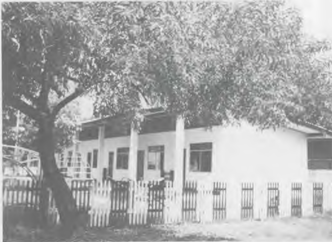
The new building of the Chiangmai Church Kindergarten which is about 50 kilometers from the Chiangmai Academy Center.
