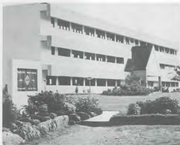
Mission College, Muak Lek Campus Administration-Classroom building
