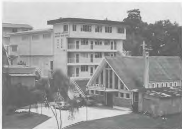
Sandakan Youth Centre with guest apartment on the top floor.
