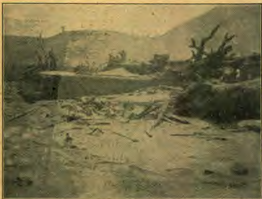
What is Left of Custom-House and Wharf.
