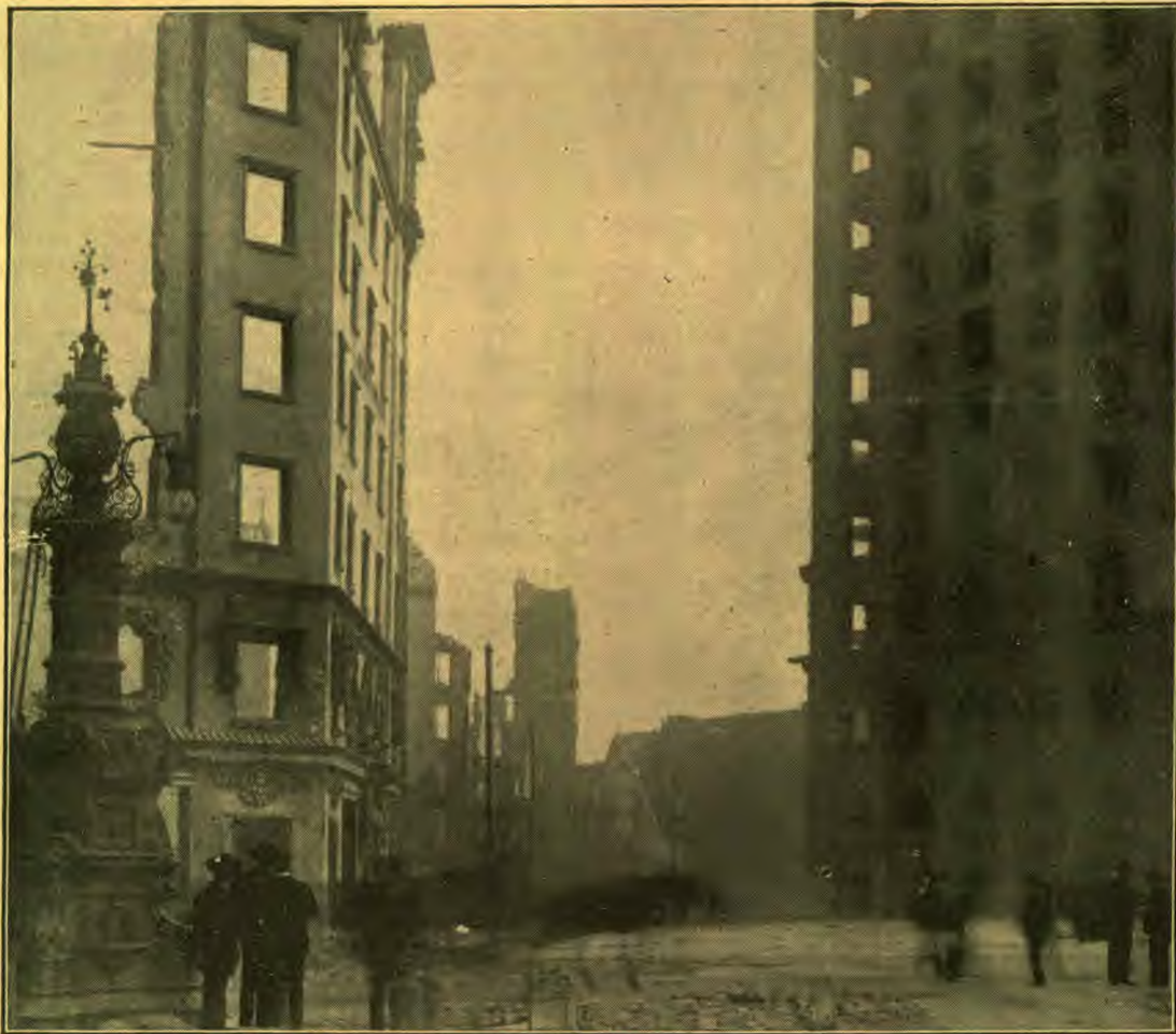
On the left side of the picture is the San Francisco Examiner Building, or what was left of it after the fire. On the right side is the Call Building. The walls stand in tact with all woodwork burned by the fire.
