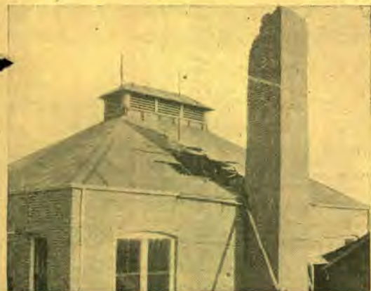
Pacific Press engine room, and broken smoke-stack which fell through the roof of the building.
