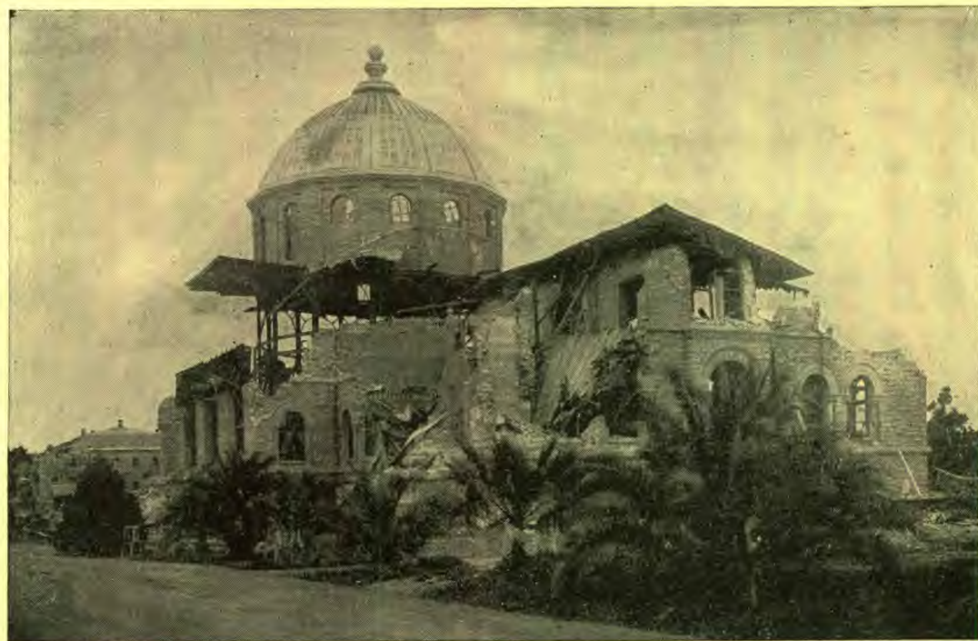
The wreck of the unfinished Library Building at Stanford University, Palo Alto, Cal., by the earthquake of April 18.
