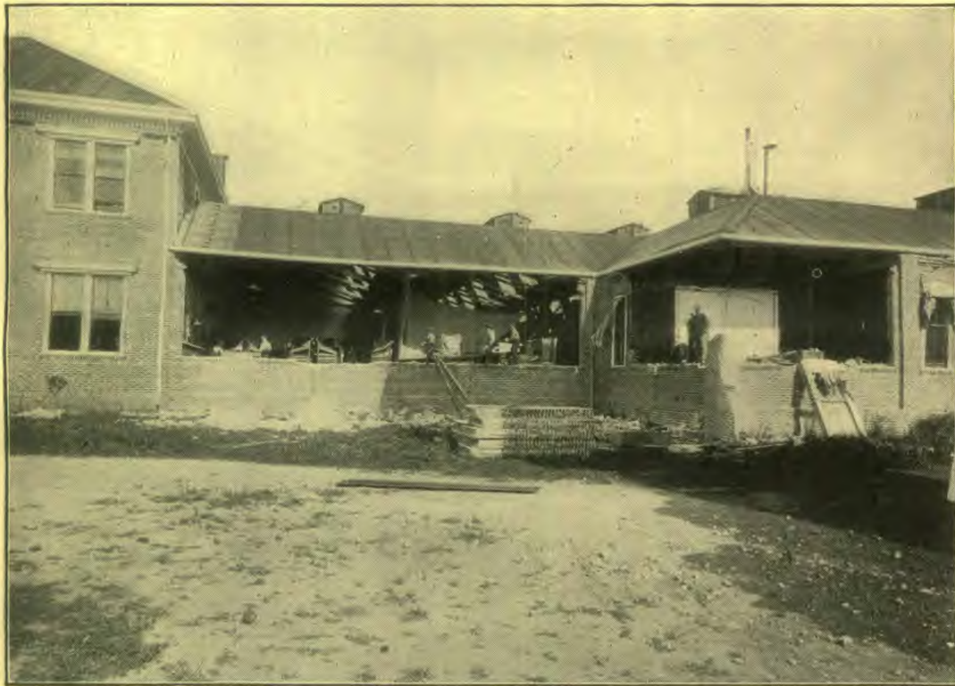
East wall of the Pacific Press Building, looking into the type room and foundry. The front wall is the only part of the outside of the structure saved.
