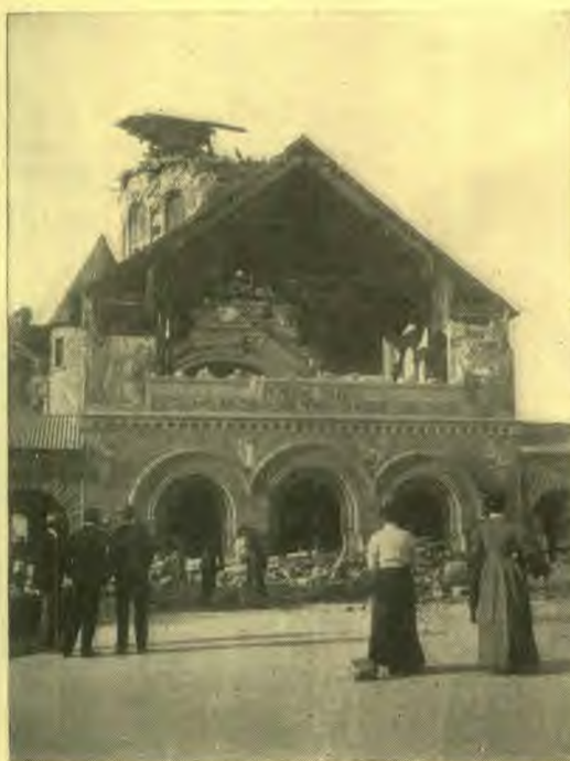
Memorial Chapel after the earthquake.
