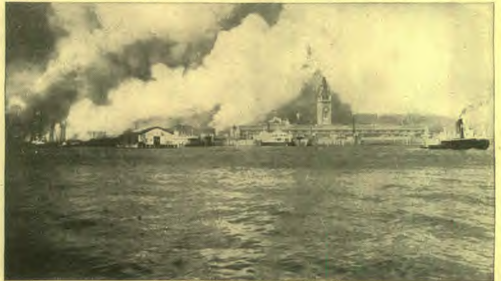
A view from the ferry-boat Berkeley on its way from Oakland to San Francisco, taken the morning of the earthquake when the fire had well started. The tall tower is the center of the Ferry Building, the fire tug at the right.
