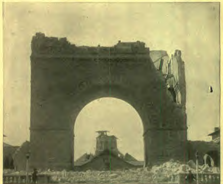
Arch at the entrance of the Quadrangle after the earthquake.
