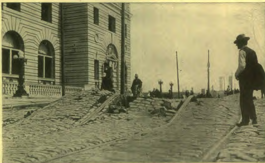
A view showing the power of the earthquake in front of the new Post Office Building, Seventh and Mission Streets. This street was previously level. The new Post Office Building was not greatly injured.
