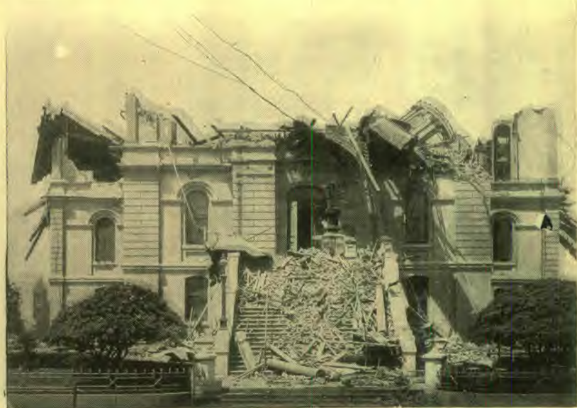
Santa Rosa Court House after the Earthquake.
