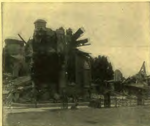
St. Patrick's Church, San Jose. Very fine structure before the earthquake, now a complete wreck.
