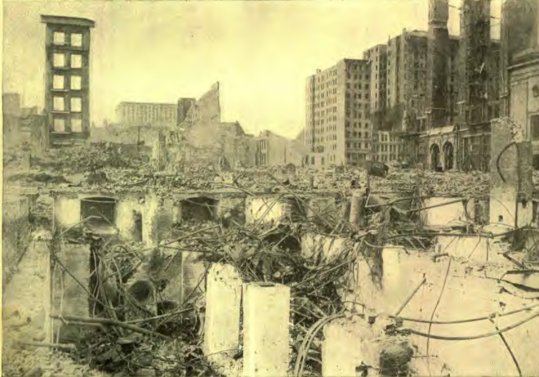
A typical wreck and tangle to be seen in the manufacturing districts of San Francisco.
