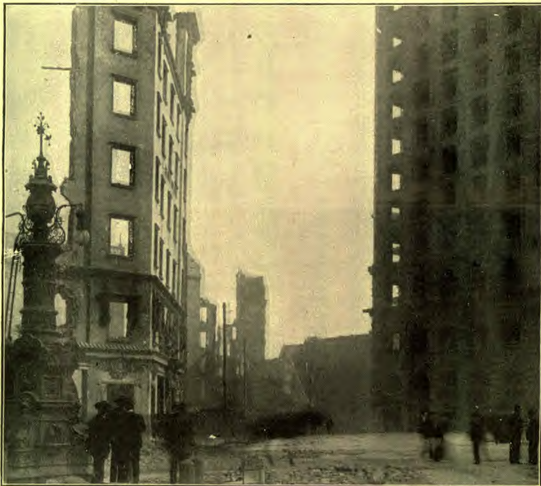
On the left side of the picture is the San Francisco Examiner Building, or what was left of it after the fire. On the right side is the Call Building. The walls stand intact with all woodwork burned by the fire.
