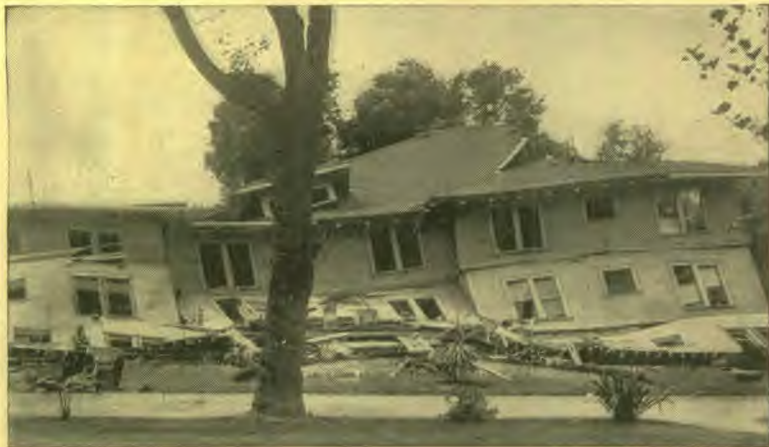
Hotel Vendome Annex. Out of this mass of wreckage 128 of the 129 occupants are said to have escaped alive. It seems an impossibility.
