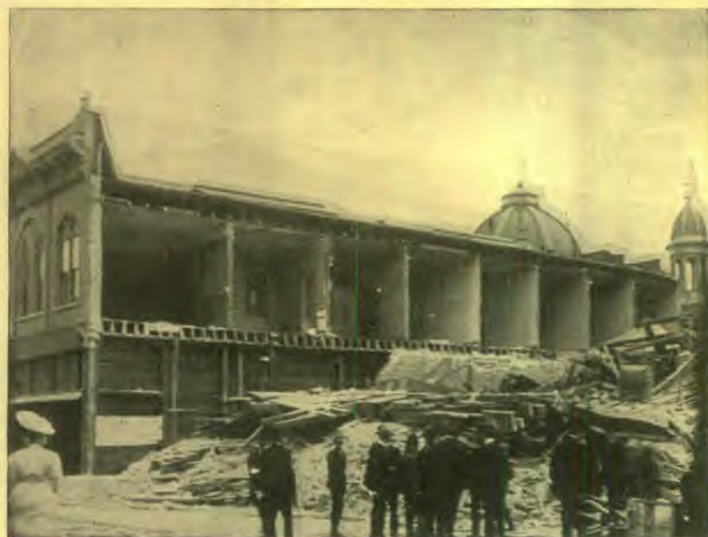
Hobson's Store—a complete wreck, under which three persons were buried. Two of these were rescued alive.
