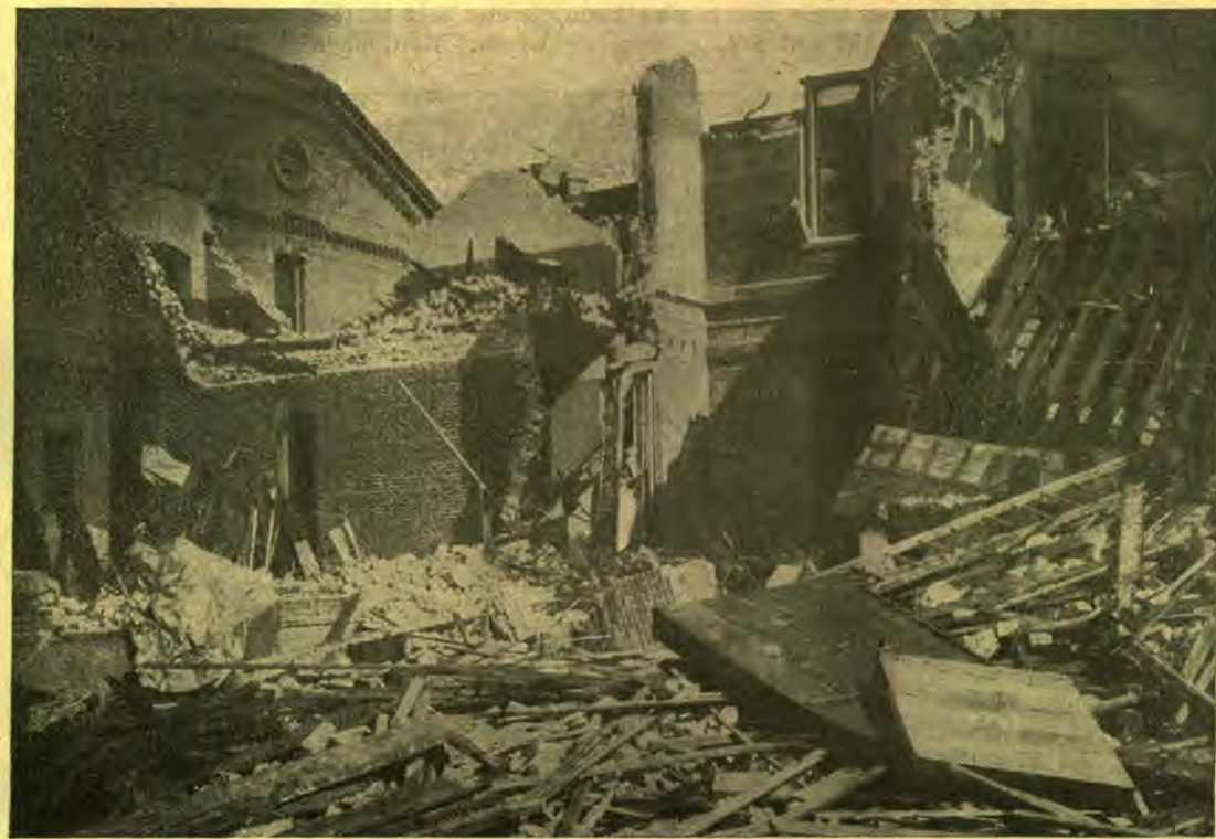
Agnews State Insane Asylum, near San Jose, showing the terrible power of the earthquake, and the utter collapse of the great building, in which 117 persons were killed. This structure was four stories, built of brick. One of the insane, a doctor, became sane.
