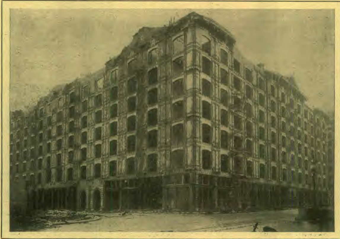
The Palace Hotel, one of the finest hotels in the world. Its register has carried the names of some of the greatest of earth's people who have passed through San Francisco. The building cost over $7,000,000, and over 30,000,000 bricks were used in its construction. Its massive walls, tied by strong bolts in every direction, withstood the earthquake shock and verified the words of the builder that "It could be shaken up, but could not be shaken down." But the fire destroyed its beauty, and left it a majestic ruin. It will be torn down, and a steel and cement structure built in its place. How uncertain are the grandest palaces of earth.
