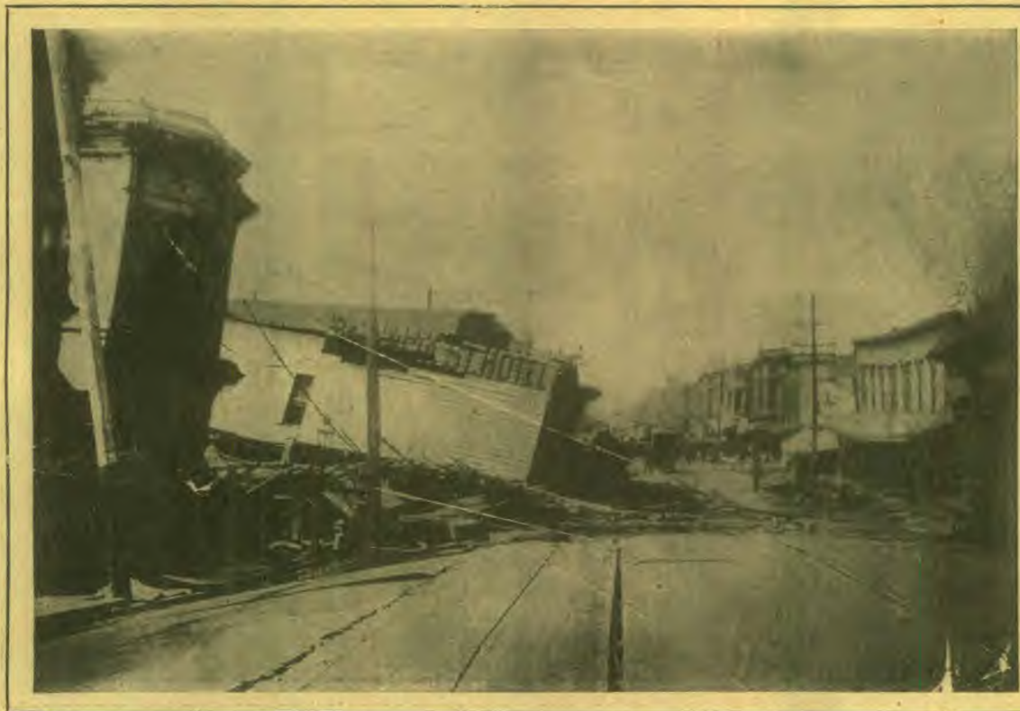
Collapse of the large, four-story Valencia Street Hotel, in which four stories were telescoped into one. The street also sunk several inches here. Between thirty and forty were killed in this building, which caught fire soon after its collapse.
