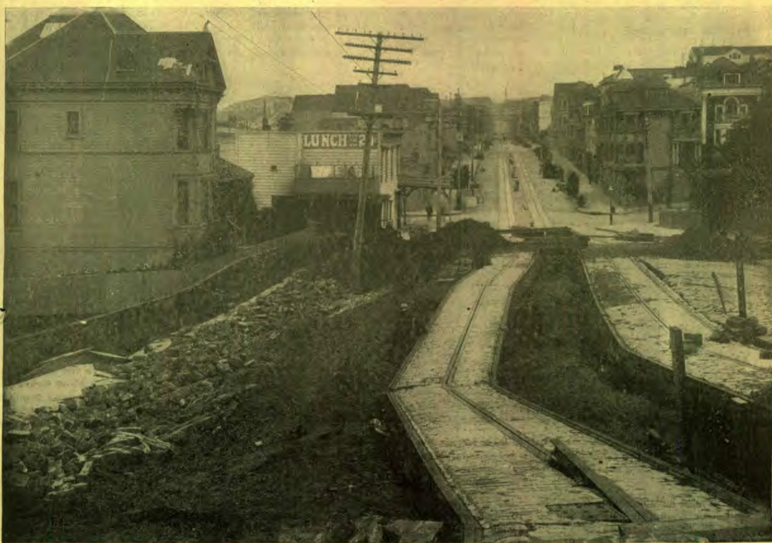
Union Street near Van Ness Avenue. This street was formerly straight, as may be seen from the track in the foreground and that in the distance forming a direct line between the two. It will be seen that the track at the left has been forced out much more than the track on the right. The depth of the cavities remaining may be seen from the men who are standing on either side of the track. This street is not on made land, but high up on the hills of northwestern San Francisco. This is one of the most striking street break-ups we have seen.
