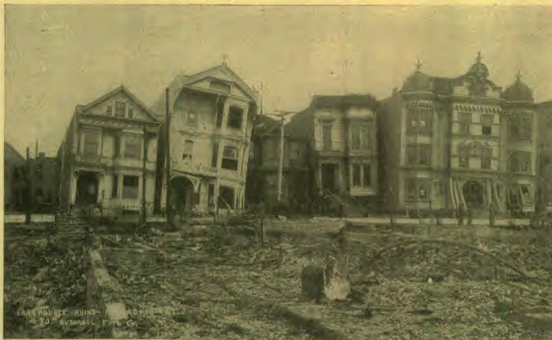
Earthquake ruins on Howard Street, between 17th and 18th. The house at the right on the corner is set over fully five feet from its foundation. This is fairly typical of the same conditions in other parts of the city. At the left of the last building standing was a house which totally collapsed, in which one woman was killed.
