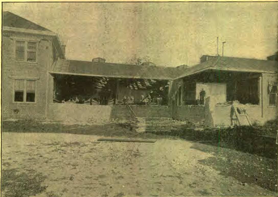
One of several wrecks in the town of Mountain View. This is the east end of the Pacific Press Publishing Company's Plant. All the wall, excepting the greater portion of the front wall, was wrecked by the earthquake, and had to be torn down. The inner supports sustained the roof.
