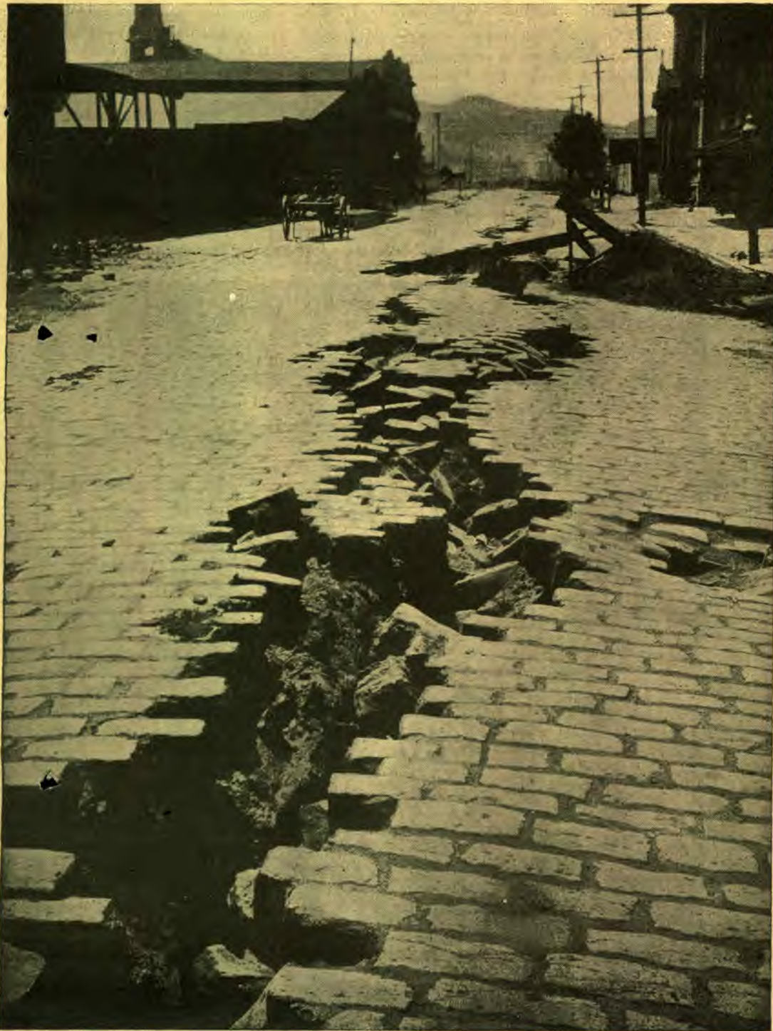
What the Earthquake did on 17th Street, near Howard, San Francisco.
