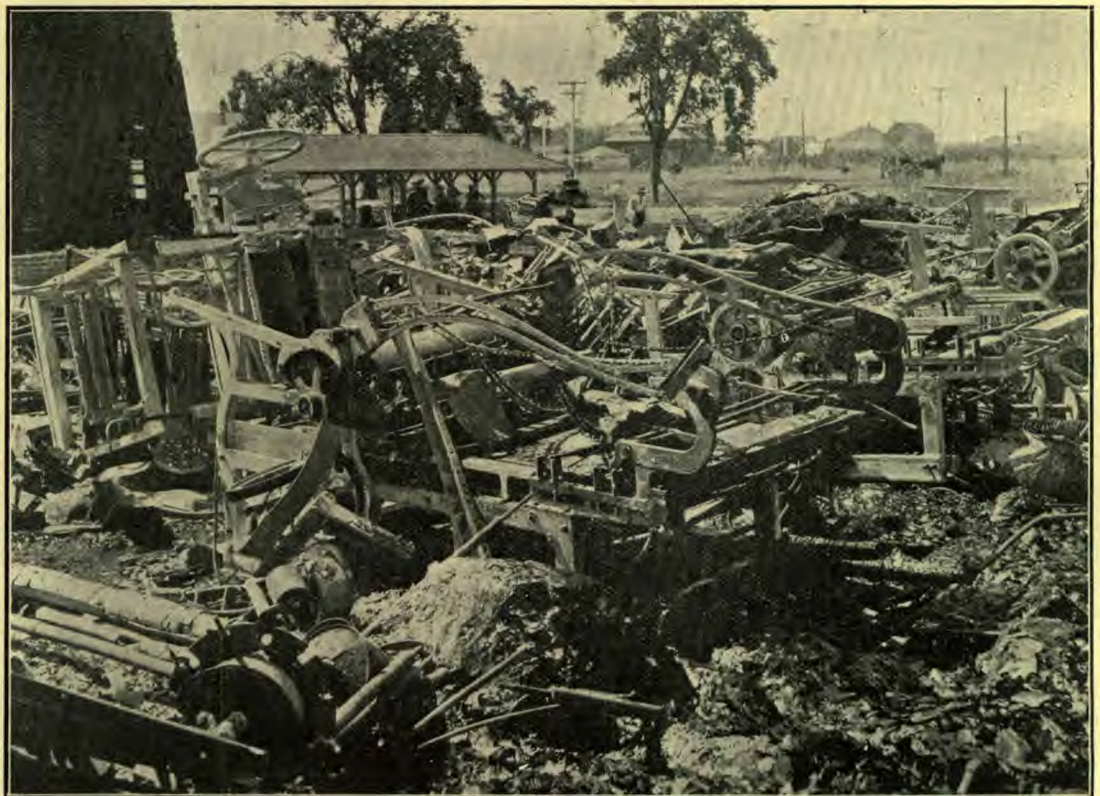
A VIEW OF THE BURNED INTERIOR.
