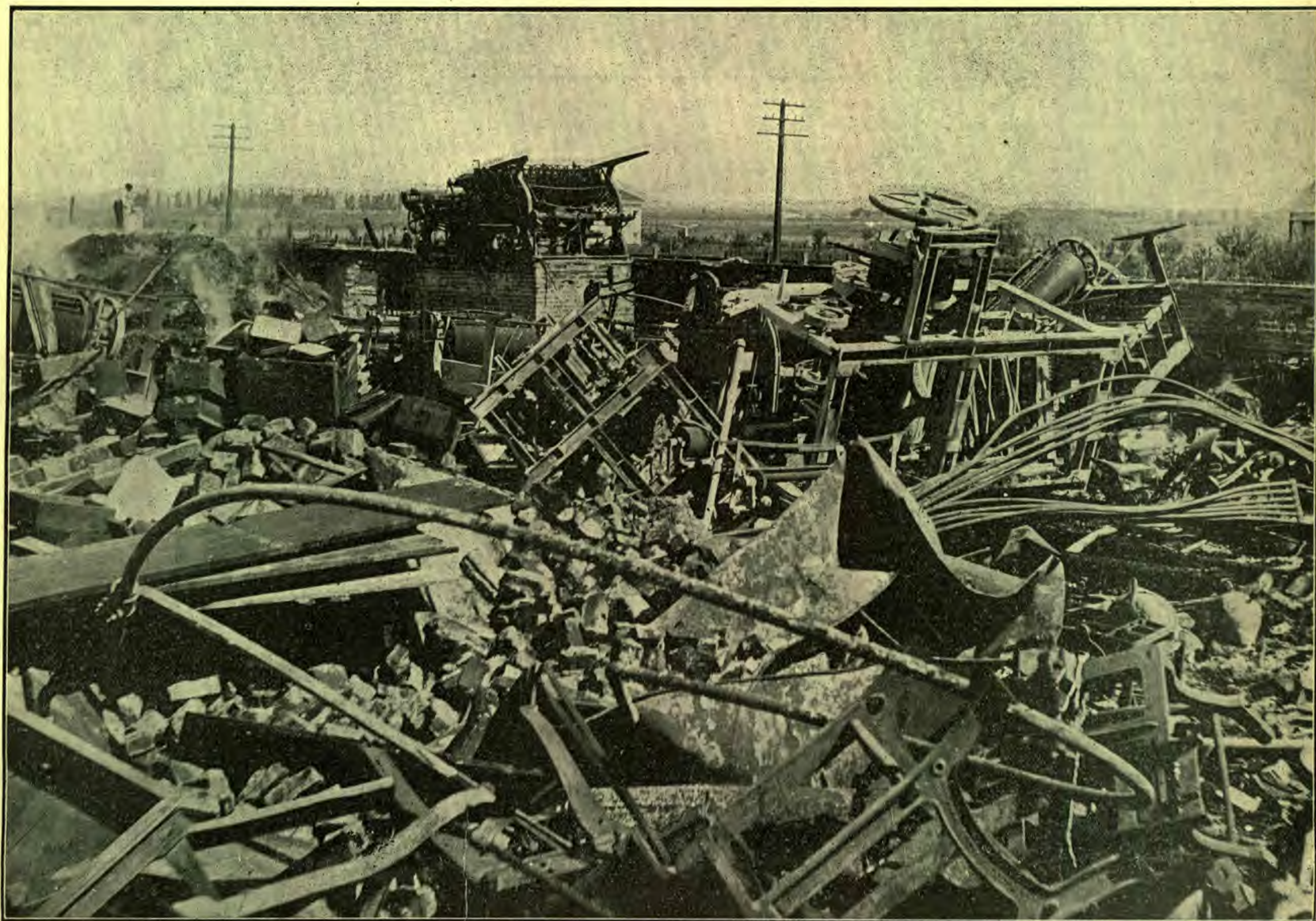
The ruins of some of the magnificent printing machines which have helped to herald the truth to the world. The press in the center background on the brick foundation is a Cottrell, which has run for twenty-five years, and was doing first-class work at the time of the fire. The large press at the right on its side is the SIGNS rotary press, installed in 1899. This issue is printed on a new Cottrell.
