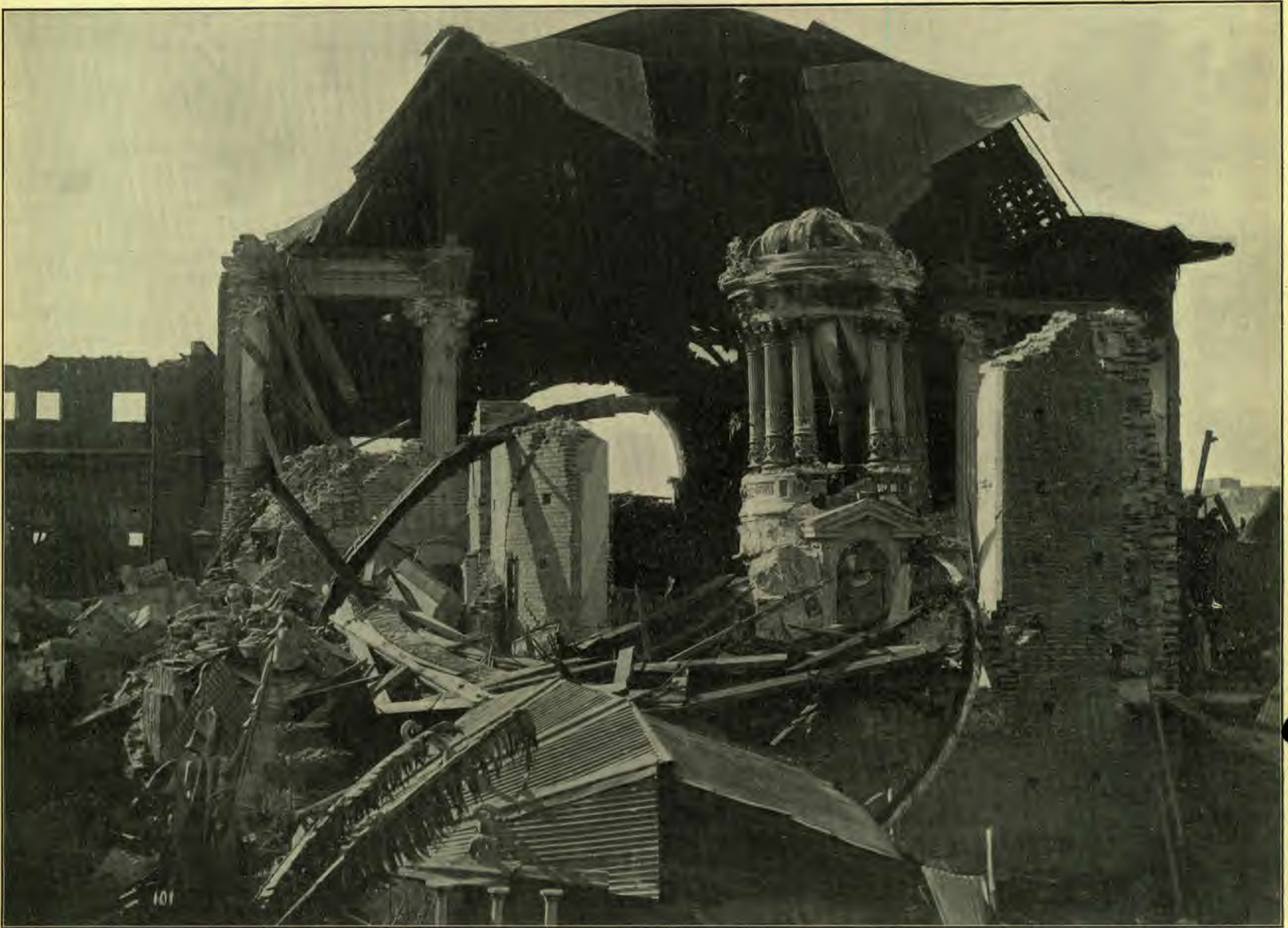
Church of Merced, Valparaiso, after the Earthquake of August 16, 1906.
