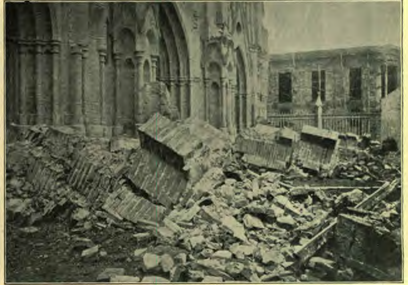
Church of Salvador, Santiago, Chile, after the Earthquake of Aug. 16, 1906.
