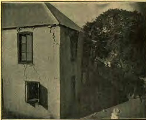
Rear View of the S. D. A. Church after the Earthquake.
