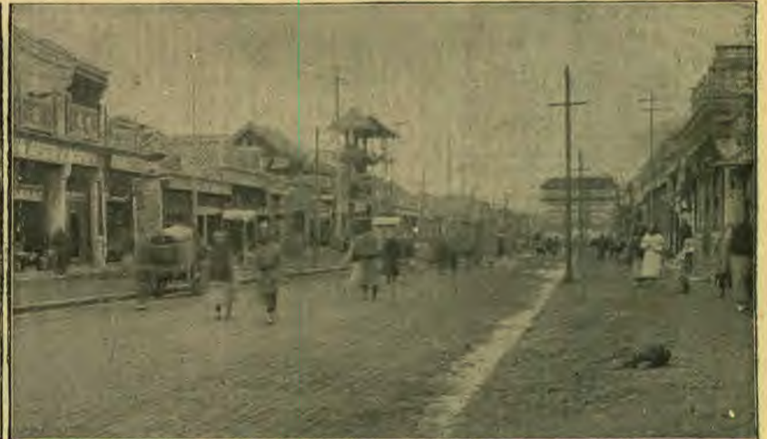
View of the Same Street at the Present Time.
