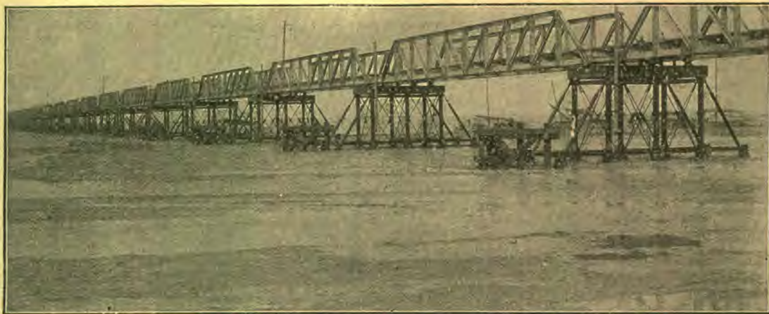
New R. R. Bridge, spanning Yellow River on the Hankow-Peking line. Length, 3,007 meters; number of piers, 103, each of 30 meters span. Built in two years by 17 Europeans. One hundred tons test.
