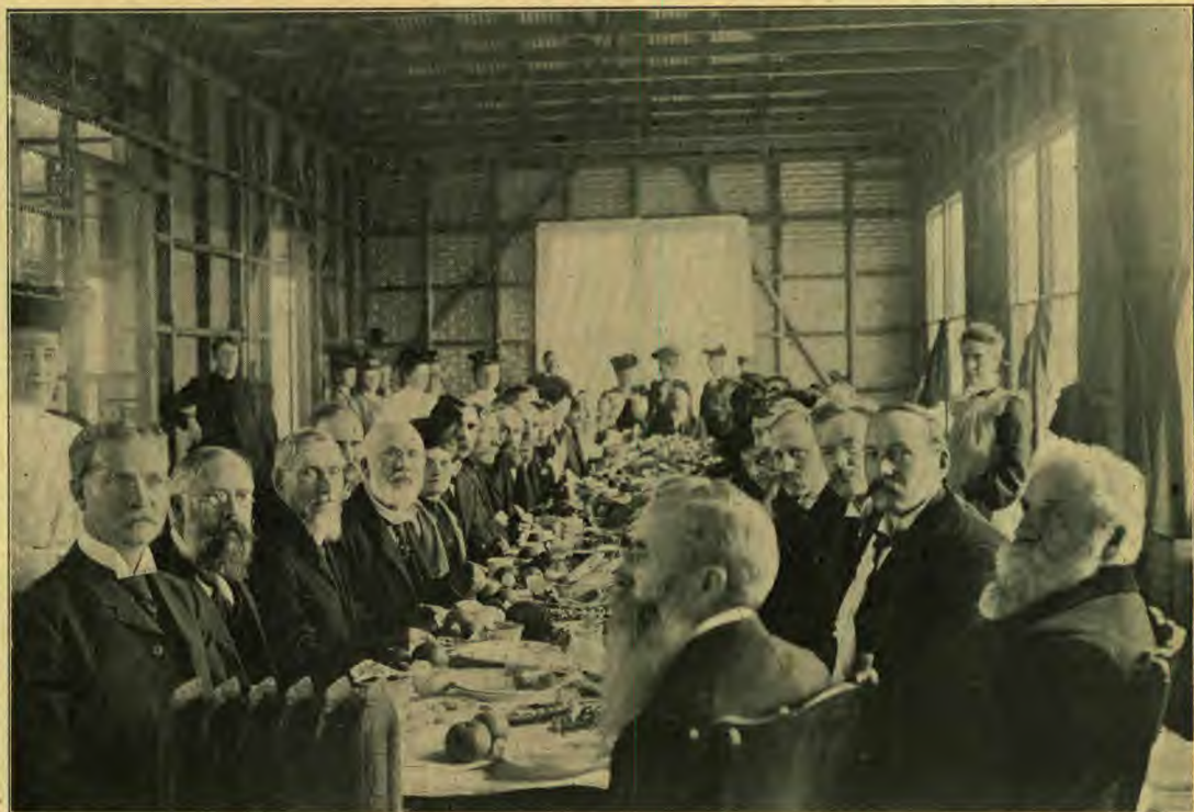
At our last stockholders' meeting, Jan. 28, 1907; lunch generously provided by the ladies of Mountain View Church. The building is now occupied, tho not quite completed. Work is more than we can do at present. Before many months the congestion will be relieved.
