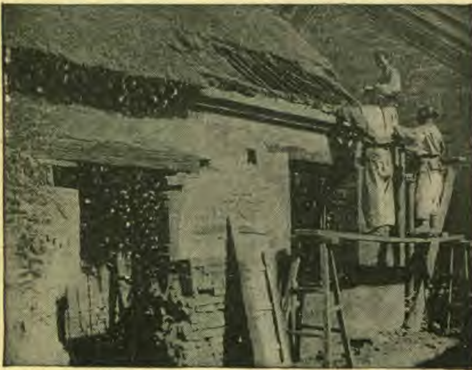
Repairing House for Mission.
