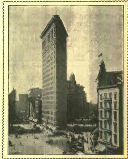
"Flat-Iron" Building, New York. Only About Half as High as the Life Insurance Building in Course of Construction.
