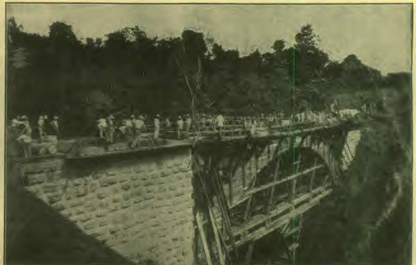
Constructing Bridge of Toa Alta-Corozal Road, Porto Rico.
