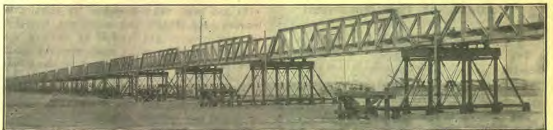
Railroad Bridge Spanning Yellow River, China. There are 103 piers, each span being about ninety feet, one hundred tons test.
