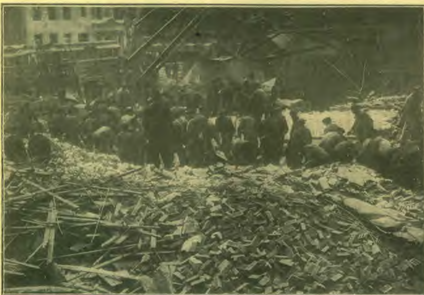
Digging for human beings alive or dead in the ruins after the explosion. The cause seems to have been the ignition of Pintsch illuminating gas mixed with air by an electric spark. The explosion followed the breaking of a gas-main under the power-house.
