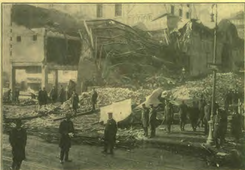
The ruins of the power-house at the Grand Central Terminal in New York, December 20, said by the "Scientific American" to be the worst at railway terminals; 10 were killed and 200 injured. The ruins show the tremendous power exerted.
