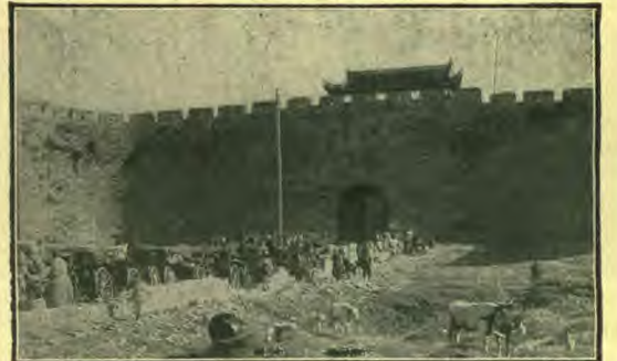
Gate leading into the city of Nanking, the old capital city of China, showing the immense height of the city walls, against which the small field-guns of the revolutionists had but little effect. These walls are from 30 to 50 feet high and 23 feet thick.
