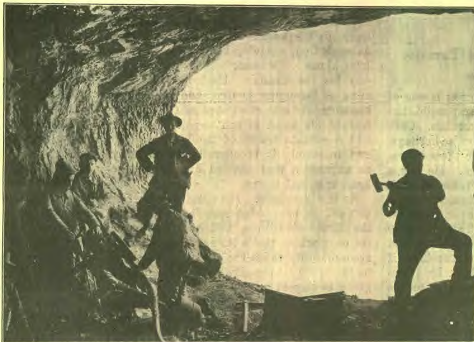
Piercing the last wall in the great Jungfrau tunnel, in Switzerland, over nine miles long. Its terminal at Jungfraujoch is 11,410 feet above sea-level. Its object is to open up for travelers some of the sublimest scenery of the Alps. The upper station lies between two great mountains, the Jungfrau, 13,672 feet high, and the Mönch, over 13,465 feet. February 21 the dynamite shot was fired which opened the tunnel. Great hotels are built at the highest station, and all winter sports may be held in midwinter.
