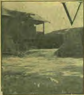
A STREET WASHED OUT IN THE SUBURBS OF LOS ANGELES. THE CONCRETE MANHOLE AT THE RIGHT WAS EVEN WITH THE SURFACE OF THE STREET, AND IS NOW A LANDMARK, SHOWING WHERE THE STREET WAS.
