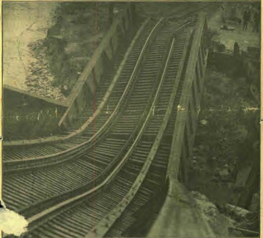
STEEL BRIDGE NEAR AVENUE 35, LOS ANGELES, WARPED BY THE FLOOD
