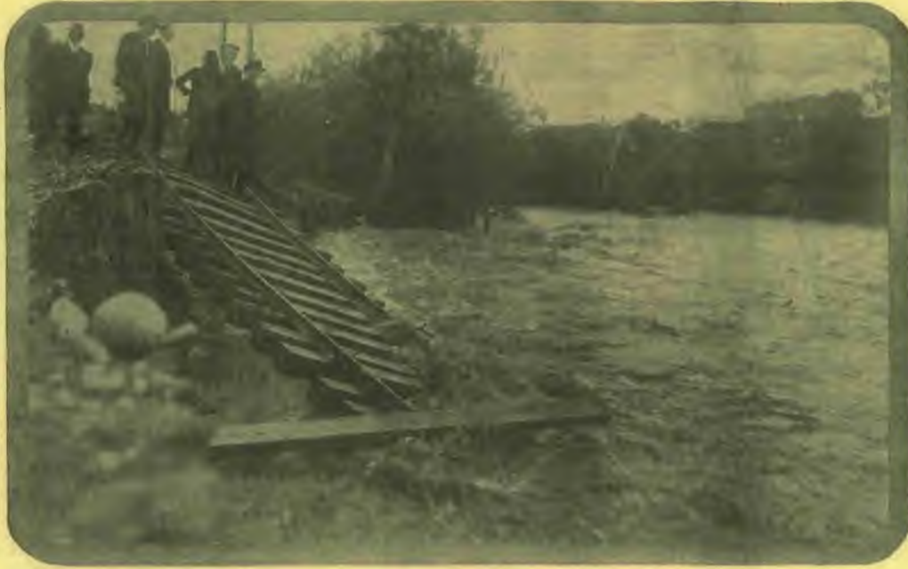
ONE OF THE MANY ELECTRIC RAILWAY BRIDGES WASHED OUT NEAR LOS ANGELES BY THE LATE STORM
