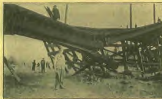
ELECTRIC RAILWAY BRIDGE AT GLENDALE BROKEN BY THE FLOOD
