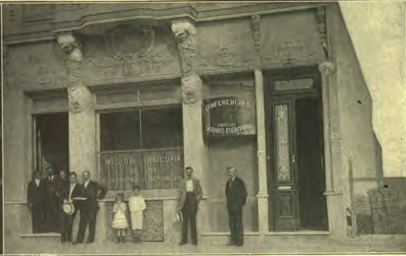
Book depository, chapel, and mission home in Montevideo, Uruguay, where the South American Union Conference was held. This building, like all the better class of structural work on the east coast, is of brick, covered with heavy cement plaster, and resembles solid concrete. It cost about $7,000, and is the best city building we have in South America.
