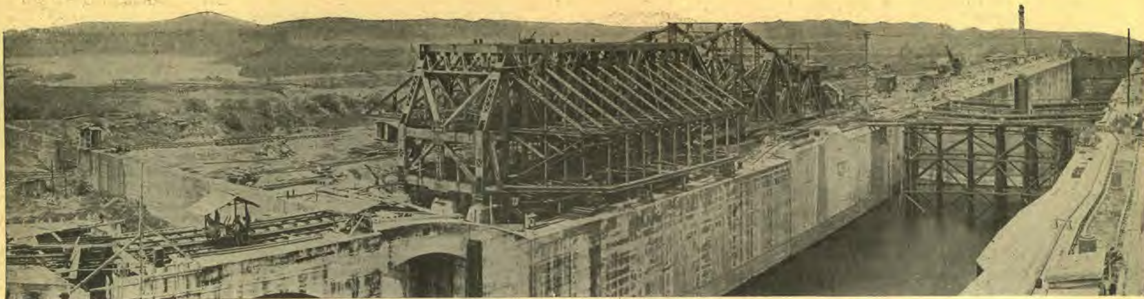
A PANORAMIC VIEW OF GATUN LOCKS, LOOKING DOWN TOWARD THE ATLANTIC OCEAN, AND The emergency dams shown at the right and left of the lock chambers may be swung across the channel, and the series of gates lowered, the
