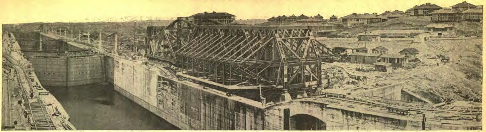
SHOWING TWO SETS OF LOCKS AND THREE SETS OF GATES AND THE EMERGENCY DAMS
