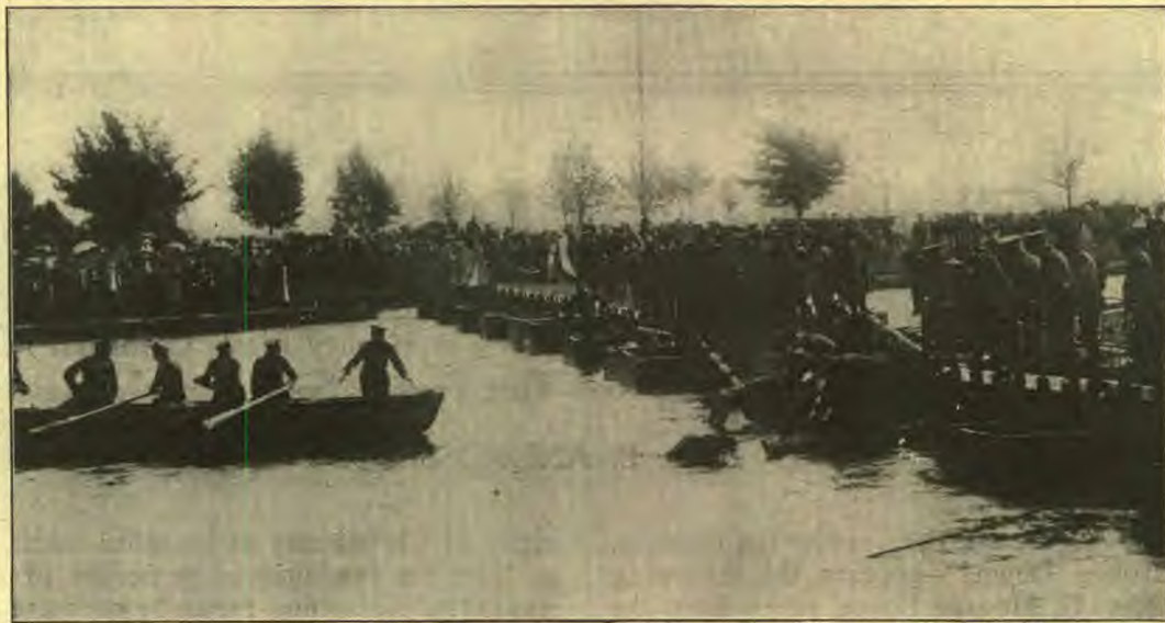
Pontoon bridge built by British engineers. The planking in a section in the center has broken down, letting two horses fall in, and the men are trying to rescue them. These pontoons are carried with the army, so that a temporary bridge can be immediately built across a stream.
