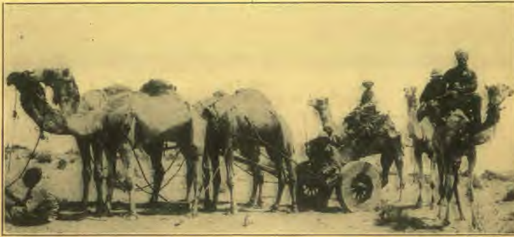
Camels draw chariot that lays telephone cable in the desert for the British forces operating in the Egyptian area.
