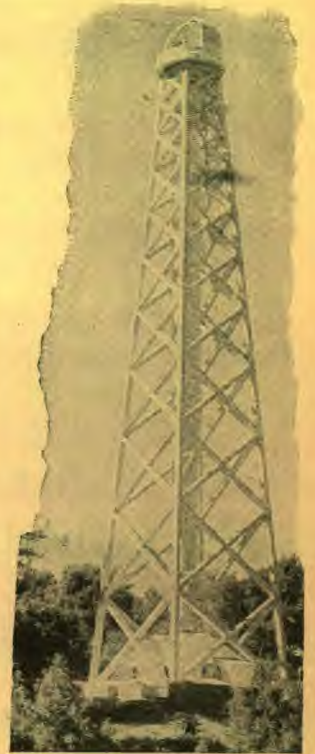
A new type of telescope, the tower telescope, which has a focal length of 150 feet.
