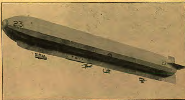
International Film A British dirigible of recent type, carrying its own aeroplane attached underneath, which marks a new advance in aviation. As the balloon leaves the ground, the pilot is already seated in his plane, ready for instant release and flight. The plane serves both for scouting and for driving off enemy aircraft.
