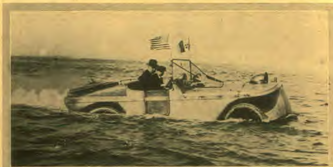
The "Sirena" is the latest amphibious monster invented by man. This particular motor car-boat is capable of making sixty miles an hour over the highways; and when it comes to a river or a lake, it just splashes out to where the propeller is under water, the driver throws in the clutch, and it starts off at twenty miles an hour through the waves. The inventors are now working on limousine and sedan models.
