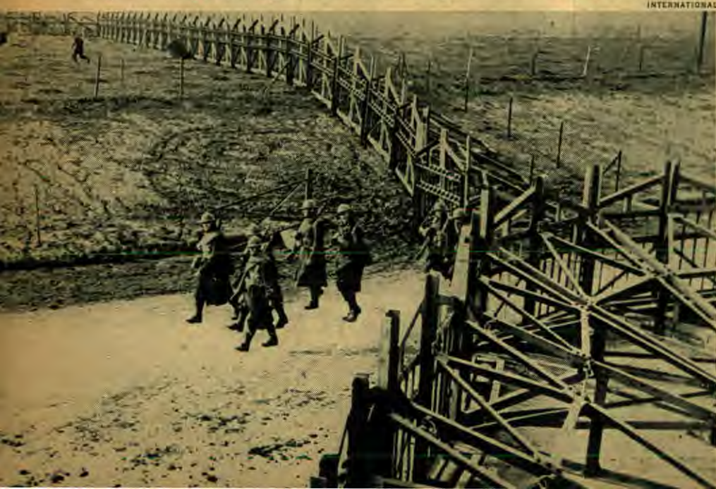
Belgium is taking no chances, and has constructed this formidable antitank fence on her border.
