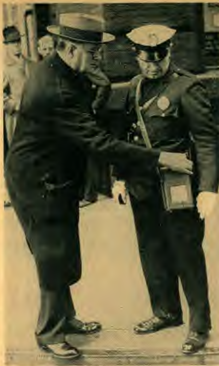
Pittsburgh police have been supplied with a new short-wave portable radio device, seen here slung over the patrolman's shoulder. The sets will be tuned in on the Pittsburgh police broadcast band, and are designed to assist in closing avenues of escape to criminals. The small square in the center of the instrument is the loud speaker.
