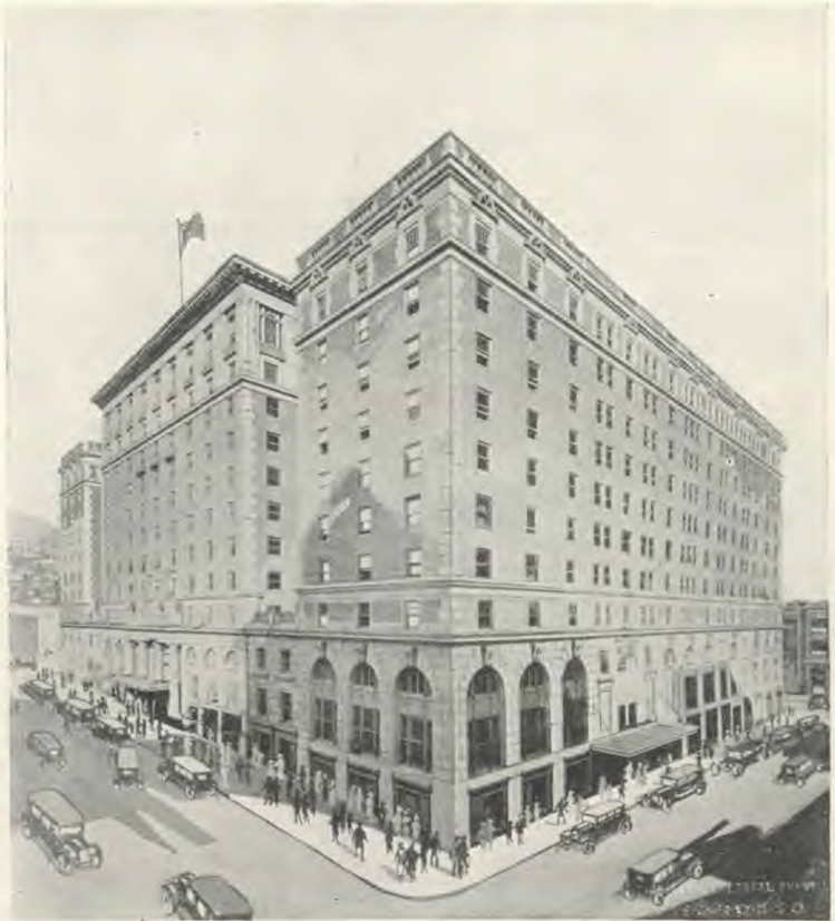
The Mount Royal, Montreal's palatial hotel, the largest in the British Empire. It is ten storeys high and covers a site 306 x 227 feet. Its electric wiring has required approximately 150 miles of wire, its telephone system is equal to the service requirements of a city of 10,000 population, and the capacity of its artesian wells is 7,200 gallons an hour.
