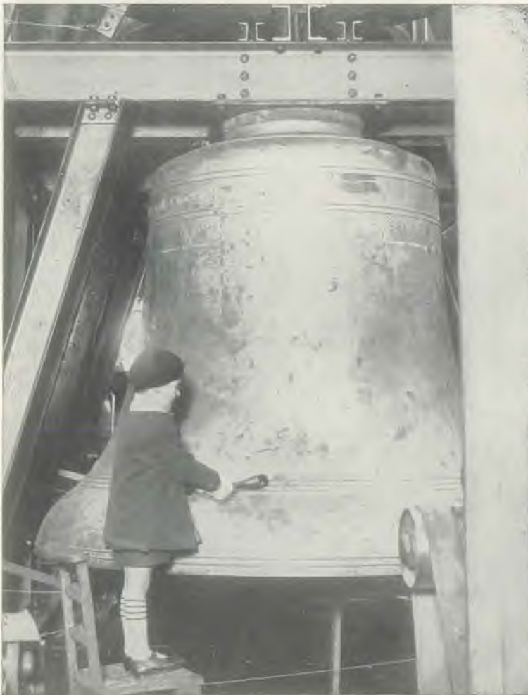
The world's greatest carillon for Victory Tower, Ottawa, is expected to ring out for the first time on July 1. The bells are from the foundries of Gillett and Johnson, Croydon, England. The carillon consists of 53 bells. The photograph shows the largest one, a bass, weighing ten tons. It has an inscription in French and English and a decoration of maple leaves around the top.
