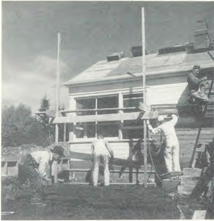
The housing shortage will be remedied. This prefabricated house was built in one day near Vancouver, B. C. Started at 9 a.m., and here shown after six hours work, it was finished at 6:30 p.m. The family moved in immediately. So, cheer up.
