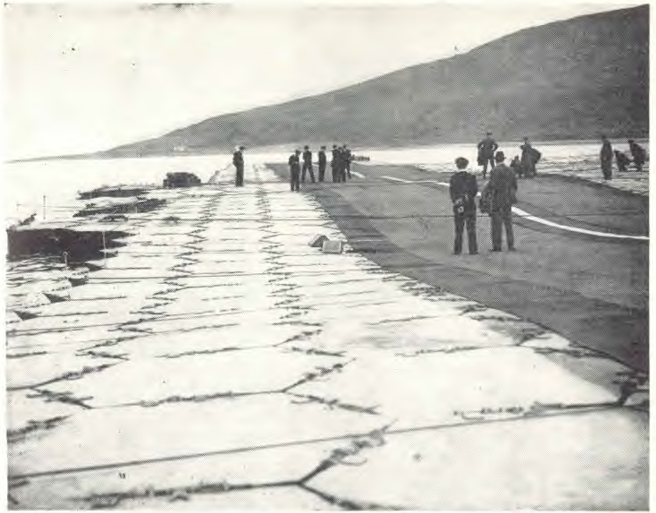
Experimenting with the "Lily", floating airstrip, for "landing" planes at sea. It undulates with the motions of the waves and the planes.
