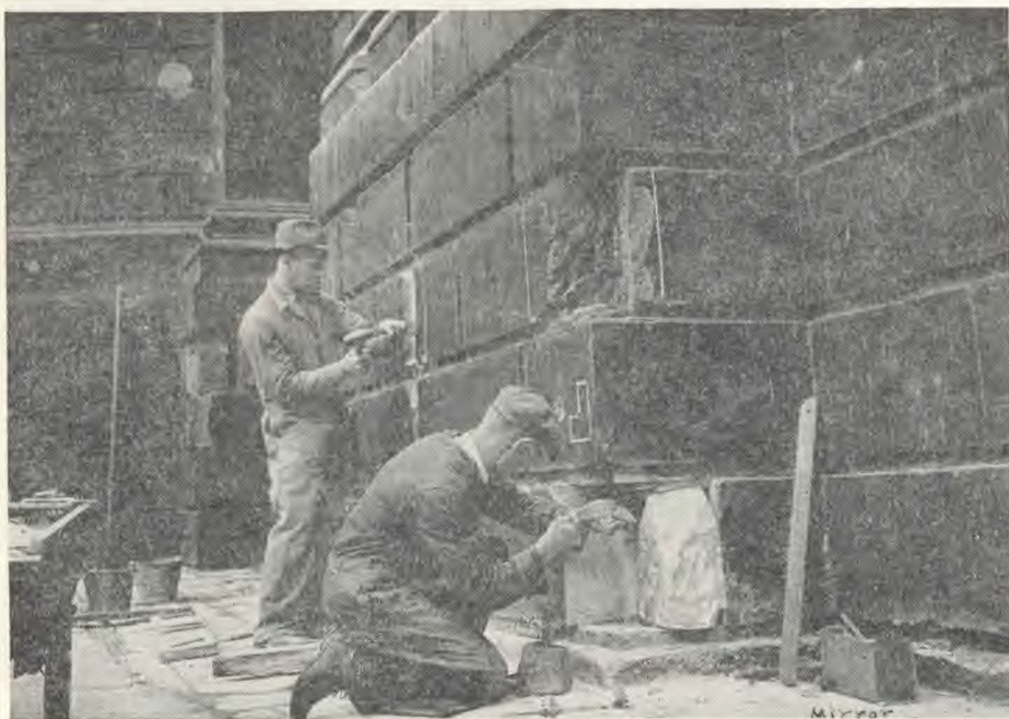
Workmen replacing bomb-chipped cornerstones of St. Paul's Cathedral, London. The gospel cornerstones have been broken in the lives of many Christians.
