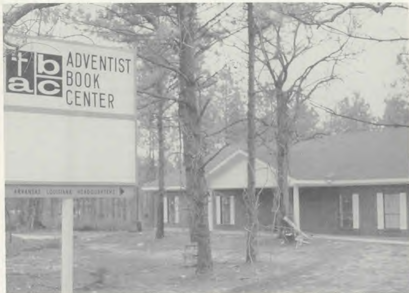
New Adventist Book Center for Arkansas-Louisiana is nearing completion.
