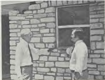
Melvin Starr and Larry Cooke inspect the walls of the new sanctuary.
