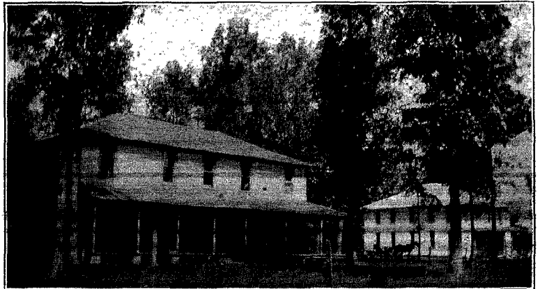
Girls' Dormitory and Academy Building
