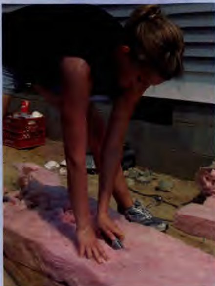
Heidi Reich from Washington state cut insulation to be installed under a Habitat for Humanity house.
