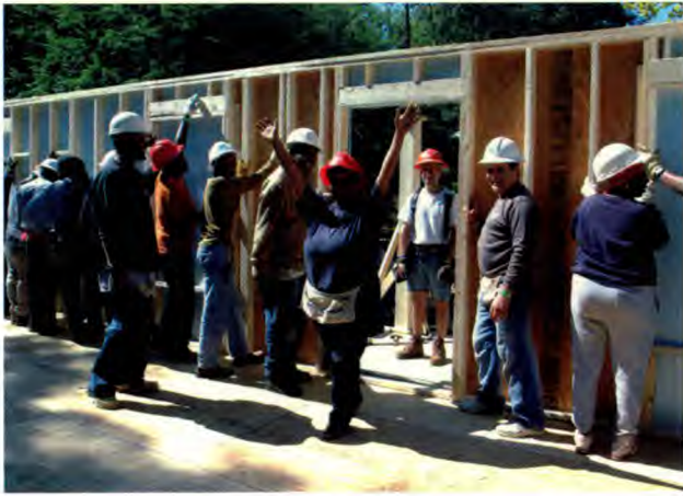
Volunteers raise the walls of the Habitat for Humanity house in Atlanta near the beginning of the project.
