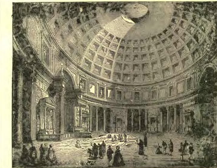
INTERIOR VIEW OF THE PANTHEON.
