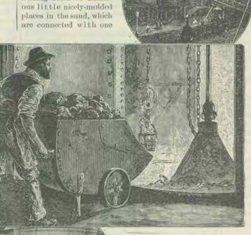
another by small duets. As the melted iron runs down this first gutter, it finds its way into all these small molds, where it remains until it is cold, when it is taken out in the shape of the pieces seen piled up in the forground of the lower part of the picture. In this shape [it is called "pig-
