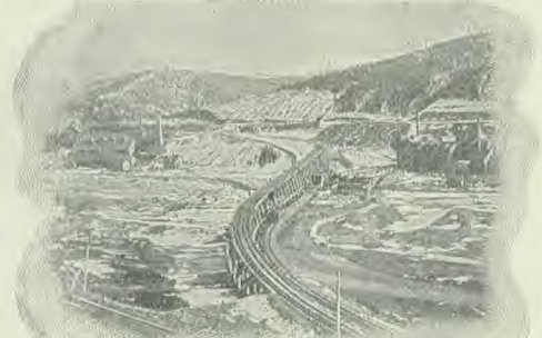
DEADWOOD CHLORINATION WORKS.
