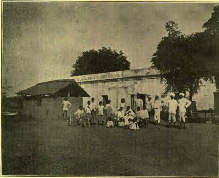
ON THE PLAYGROUND AT KARMATAR
