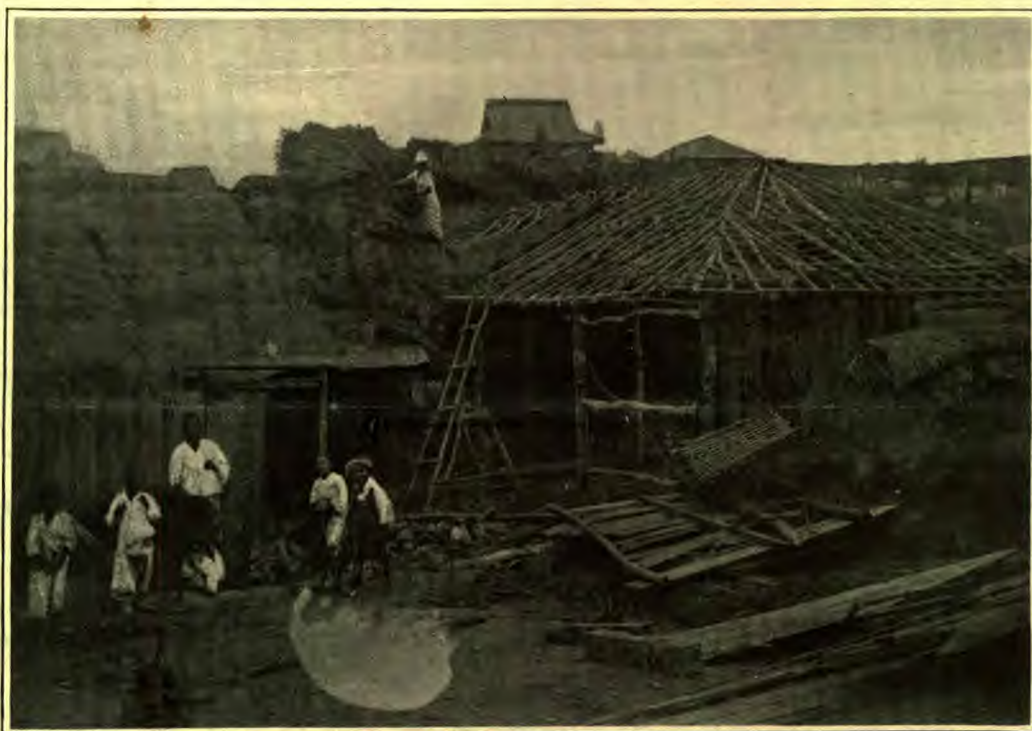
A KOREAN HOUSE — STRIPPED TO SHOW THE FRAME
