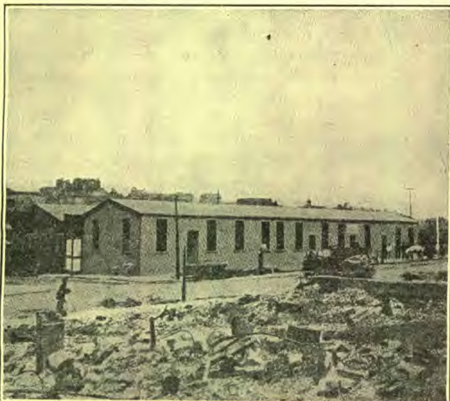
PRESENT HEADQUARTERS OF THE BOARD OF EDUCATION AND SUPERINTENDENT OF SCHOOLS, SAN FRANCISCO
